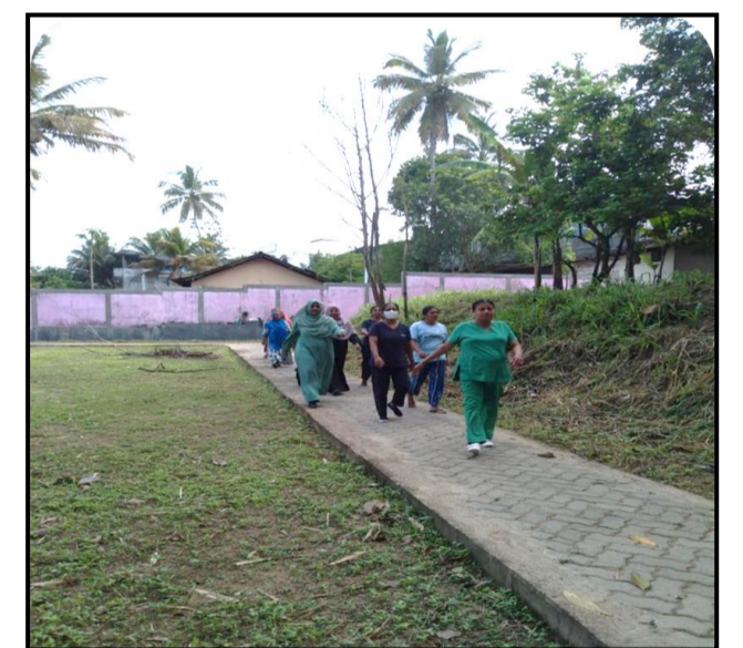
Jogging track constructed by FFC PMCU Thihariya
